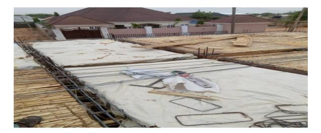
Figure 4. Laying of polythene sheets on soffit.
