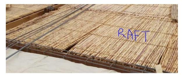
Figure 1. Sorghum raft placed as soffit in suspended slab construction.
