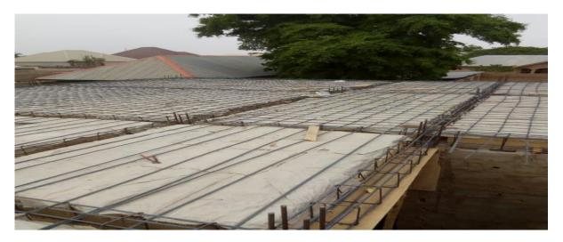
Figure 5. Arrangement of reinforcements on soffit formwork.
