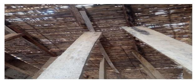
Figure 2. Underside of sorghum stalk soffit.
