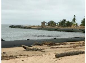
Fig. 4 Sand Tubes for Erosion Control (Source: Author's Photograph)
