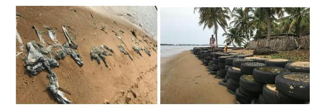
Fig. 6 The Jute Sacs for Erosion Protection Failed (Source: Author's Photograph) Fig. 7: Car Tyres Filled with Concrete (Source: Author's Photograph)
